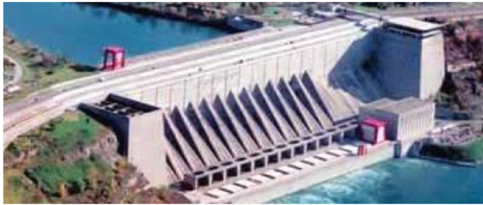
Niagara Power Project (2,441 MW)
